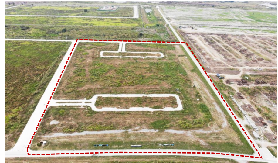
Land Development : 100% Completed
